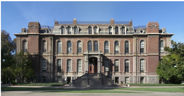
Figure: South Hall - UC Berkeley (built 1873)
