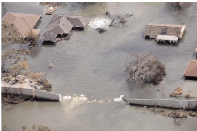
A broken levee on the east side of the London Avenue Canal in the Gentilly neighborhood of New Orleans, 11 September 2005.
